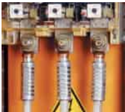
The perfect solution for transitions from aluminum to copper conductors and vice versa.
